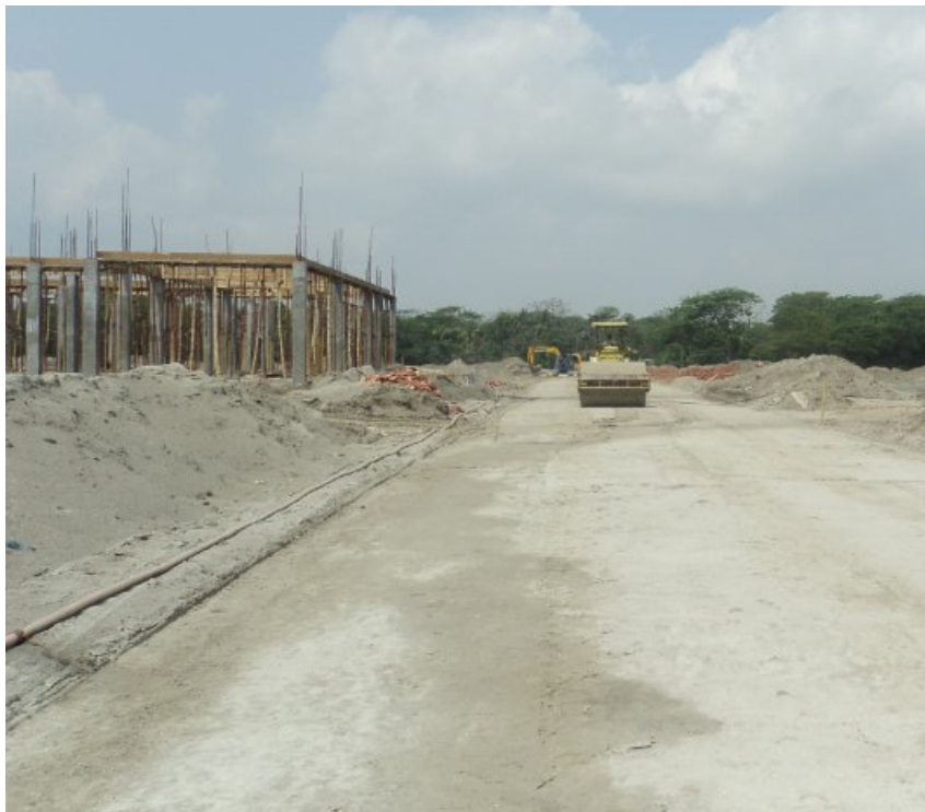
Photo No.6: Internal road construction at Jashaldia Site
