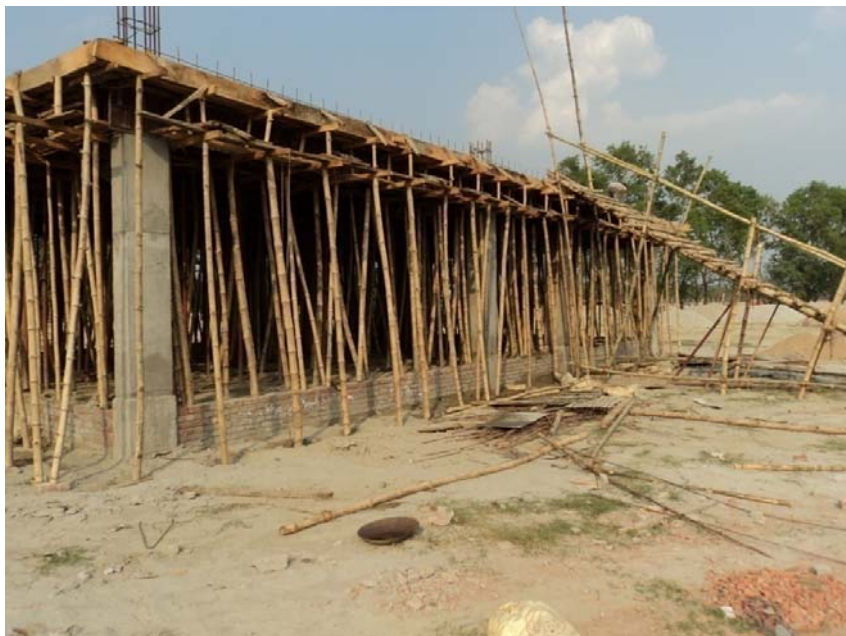
Photo No.4: Construction work of health centre at Naodaba RS
